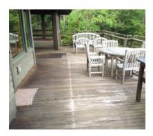
Located in the heart of Vermont's Green Mountains, this slope-side ipe deck hadn't been maintained since its installation 14 years ago. Note the drip line underneath the eaves.
